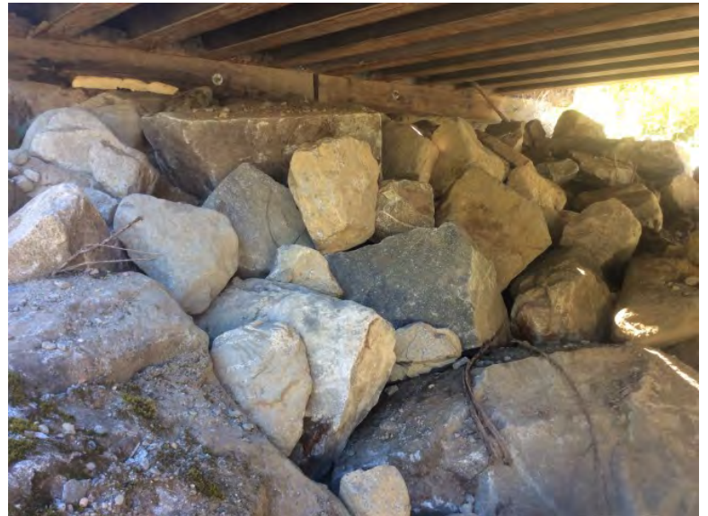
Left Bank Abutment when facing downstream
