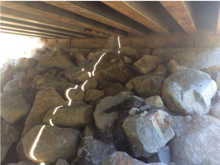
Right Bank Abutment when facing downstream
