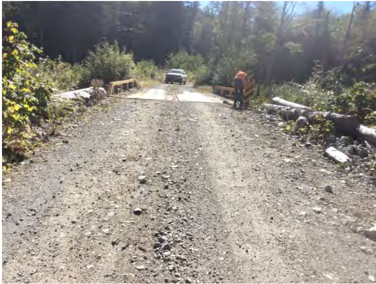
Approach from Right Bank when facing downstream
